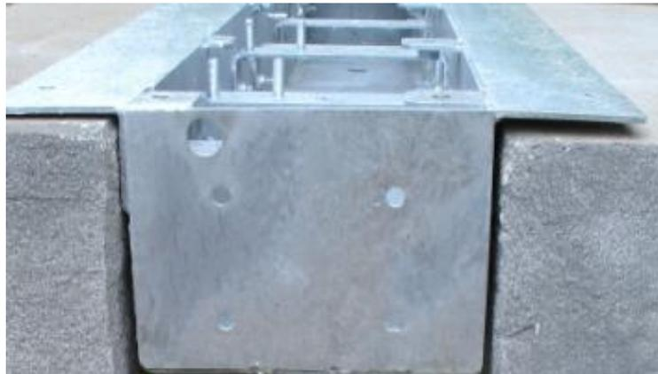
If the road surface is uneven, a layer of silicone/mortar may be applied to the area under the edges of the galvanized frame prior to the frame being tightened down to the roadway(to prevent vibration).
